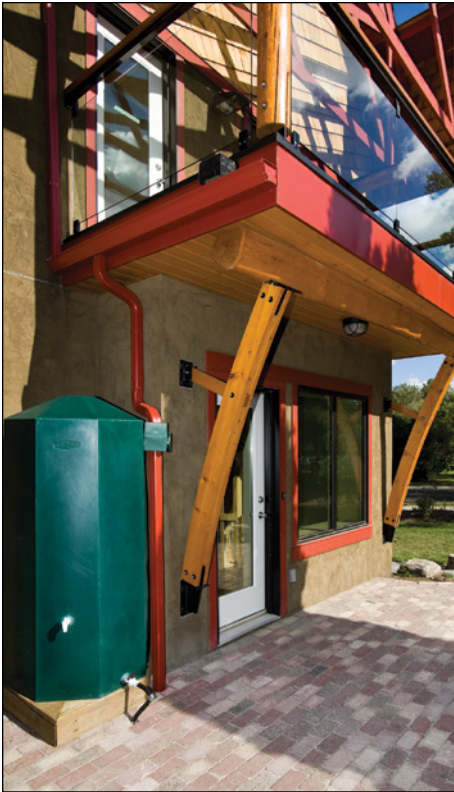
Figure 4 Rainwater harvesting at its simplest: a rain barrel placed below a downspout
